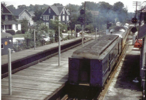
The "Scoot," with its mail car, leaves Babylon Station for Patchogue, where the mail will be unloaded and the car returned west. LIRR carried mail until 1965, when its contract ended and all mail cars on the railroad, including this one, were scrapped. Note the sooty roofs of the mail car and RDCs. ( Malcolm Young photo )
