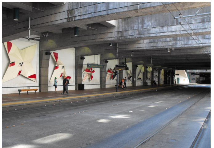
Opened in 1990, the Downtown Seattle Transit Tunnel (DSTT) has encountered controversy through its existence, from construction issues that would result in expensive retrofitting to accommodate LRVs to the use of South African granite, banned due to apartheid sanctions in the 1980s. Despite this, the tunnel has been a resounding success. Seen here is the International District/Chinatown station, opened in 1990 for buses and now also used by Central Link.
