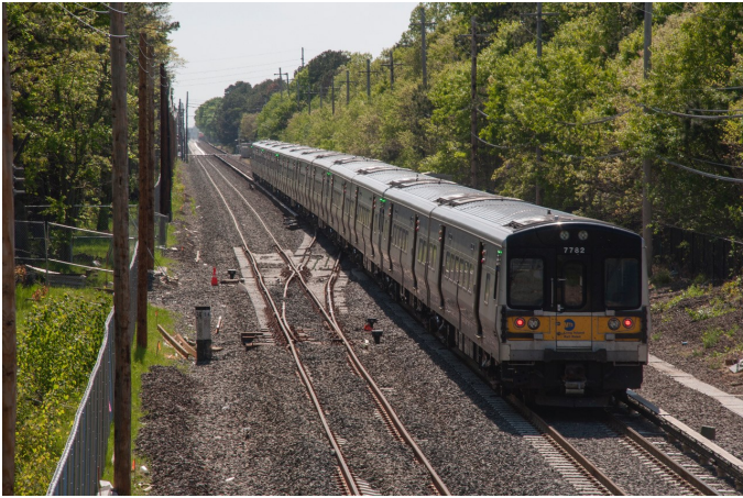
Train #2057 heading west through the future Danah Interlocking on May 21, 2018. The second track still lacks third rail and none of the four new signals have been installed yet.
