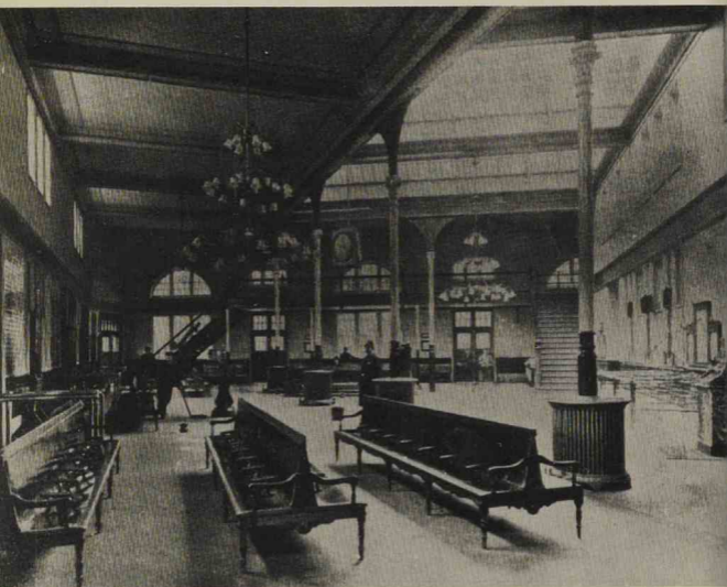
Front of the Long Island City station on 2nd Street as it looked after rebuilding in May 1903. (Eagle) (Top)
