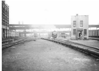
Yard Office, west elevation
