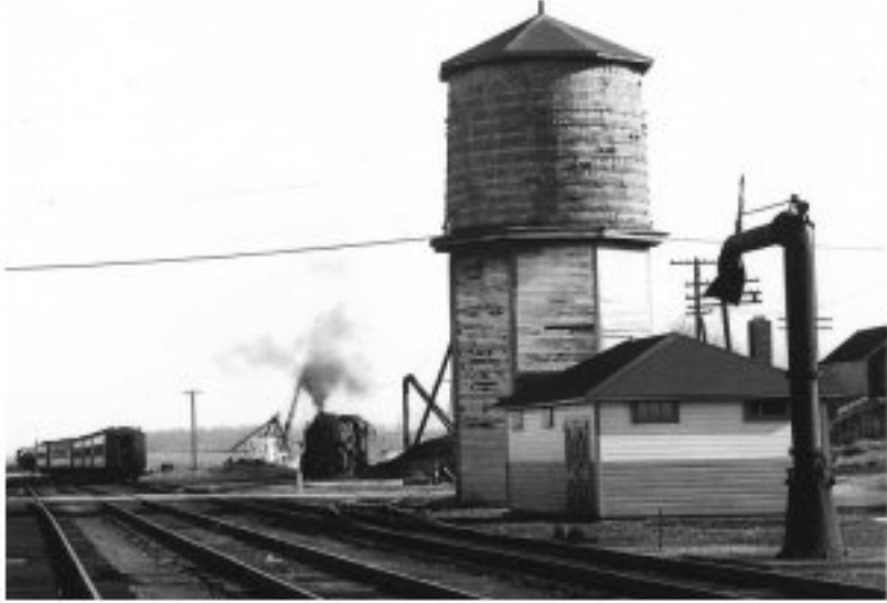
Greenport water tank - View E Section house, and water plug 2/1950 Archive: Mike Boland
