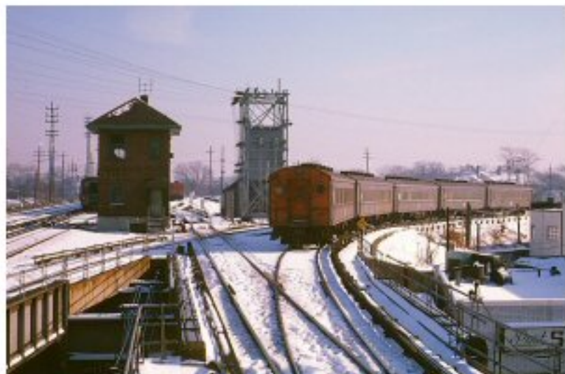
VALLEY Tower - View E Far Rockaway Branch at right Photo/Archive: Brad Phillips
