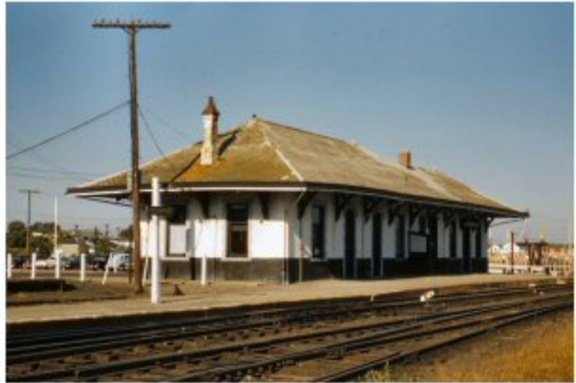
Greenport Station View NE c.1959 Archive: Dave Keller
