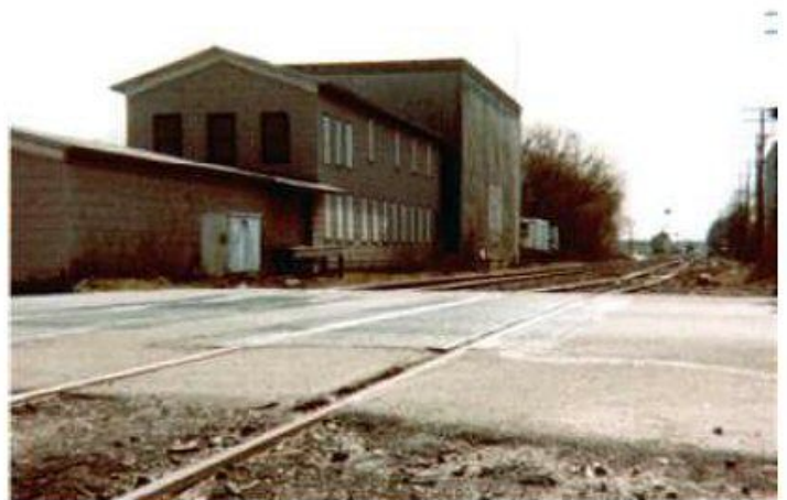
Ex-Knickerbocker Ice Co./Hiscox Chemical Works-Rider Ave., view looking west, 1996. Abandoned siding 1963. Photo/Archive: Steven Lynch
