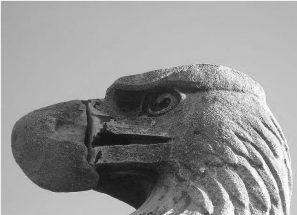
Close up view of the deteriorated beak - summer 2009
