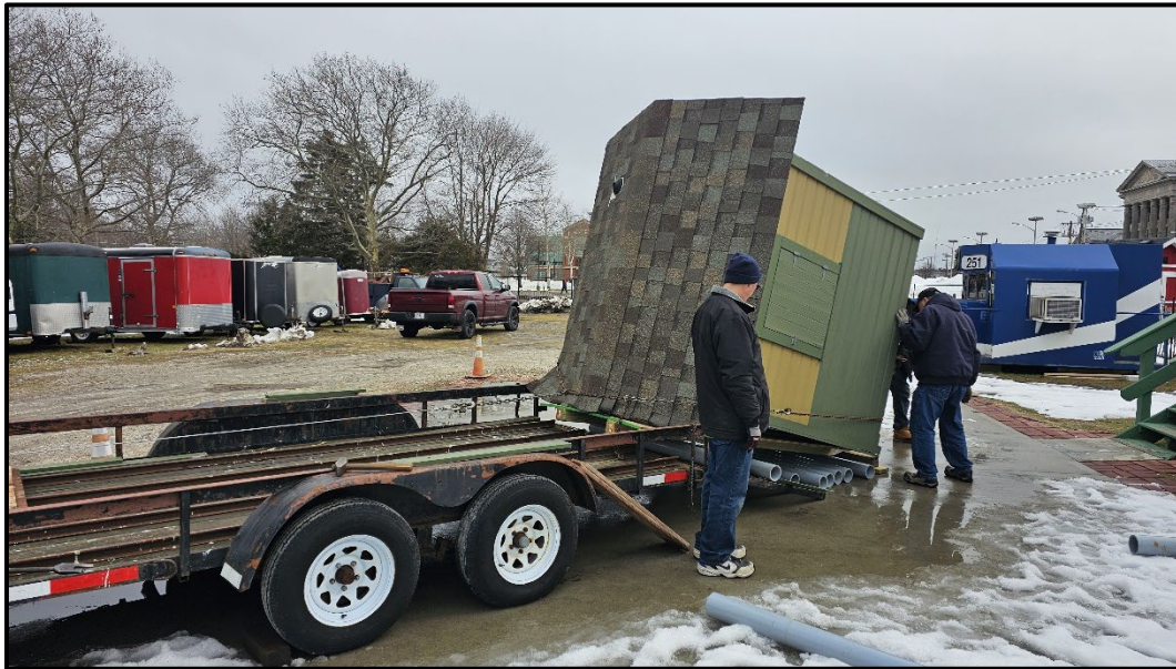
Reversing the process of using rollers to get the shanty onto the trailer, it was rolled off the trailer at the Riverhead site.
