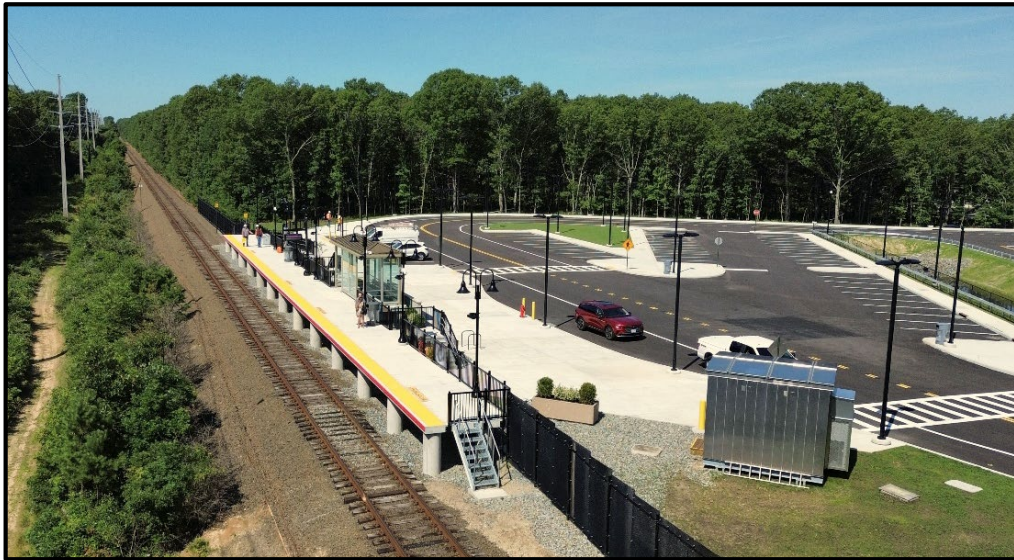
The new Yaphank – Brookhaven National Laboratories (“BNL”) station at MP 61.7 opened on July 17, 2026, this image was taken on July 20, 2026, by Barry Johnson, LIRR Road Foreman of Engines. The old station and YA Block Limit Station were located at milepost 58.6, approximately three miles west of the old facility. Chapter Vice President Bob Myers (a retired LIRR Transportation Manager) points out that an eastbound train needs a ‘K’ Clearance Card to pass YA and reach the new station. It is hoped that the car park and bus turning loop available at this site will encourage greater use of the train.
